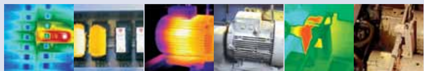
Electrical: Hot Fuses
